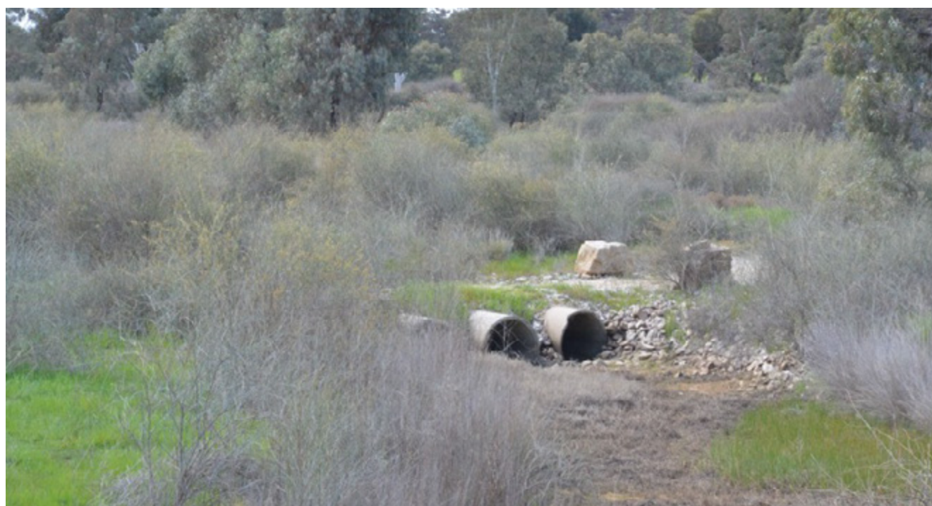
Figure 9: Culvert on Bullock Creek
