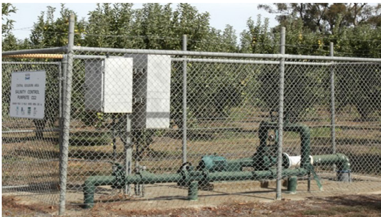
Figure 7: GMW salinity control groundwater pump
