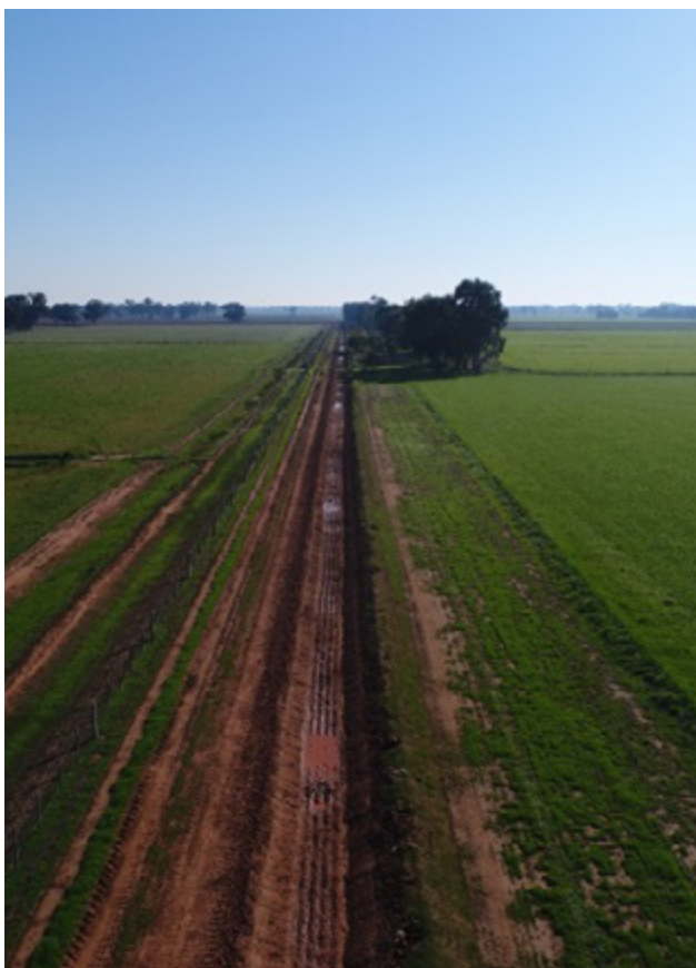
Figure 4: GMW community surface drain construction
